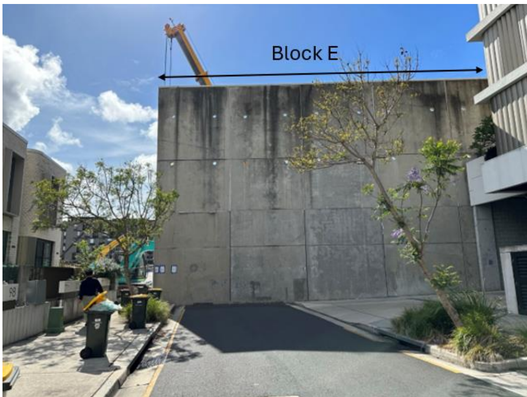
Figure 3: Site viewed from Metters Street looking east
