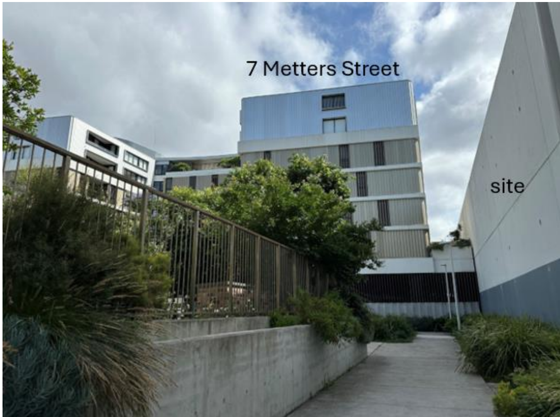
Figure 6: Pedestrian link between subject site and 74 Macdonald Street looking north to rear of 7 Metters Street
