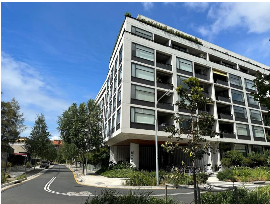
Figure 10: 5 Hadfields Street, south-west of the subject site
