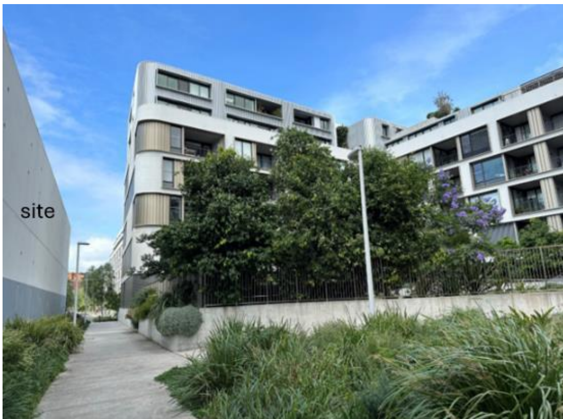
Figure 7: Pedestrian link between subject site and 74 Macdonald Street looking south
